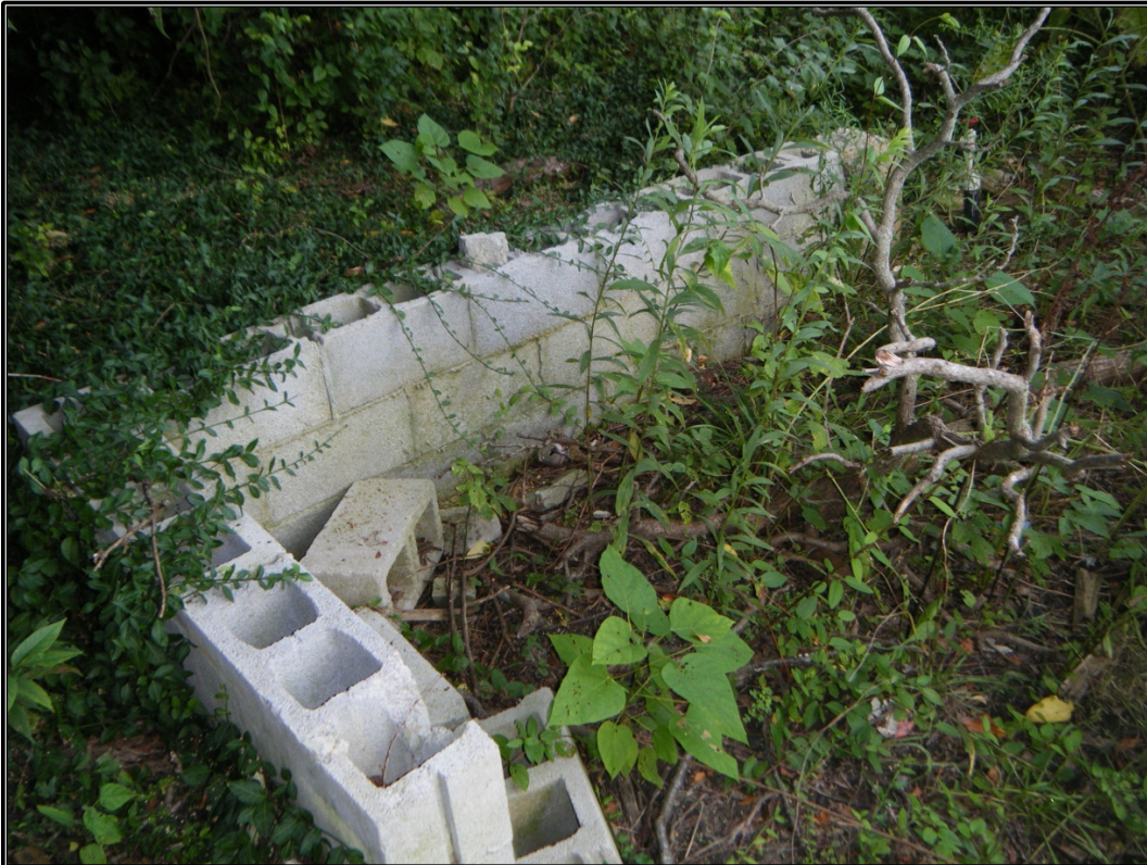
Figure 16. Feature 2: L-shaped foundation outline, facing north.
