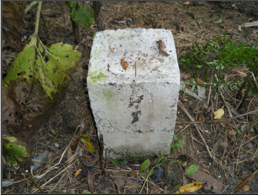
Figure 17. Feature 2: foundation piers.
