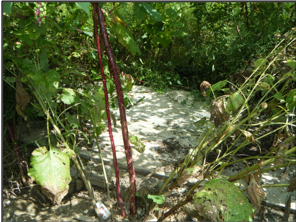
Figure 18. Feature 2: foundation pad, facing north.
