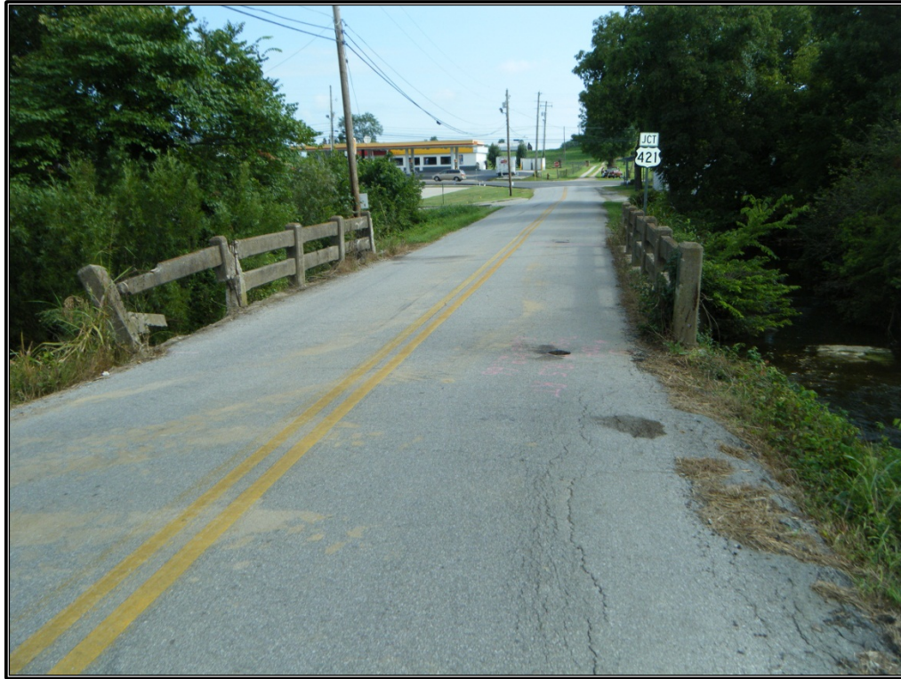
Figure 6. Standing KY 3376 bridge that spans Hays Fork, facing northeast.
